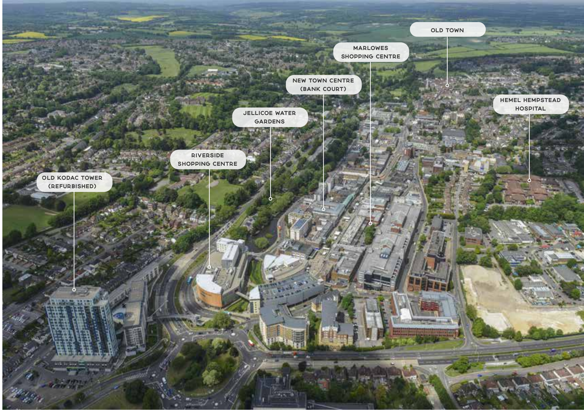
aerial view of Hemel Town Centre
