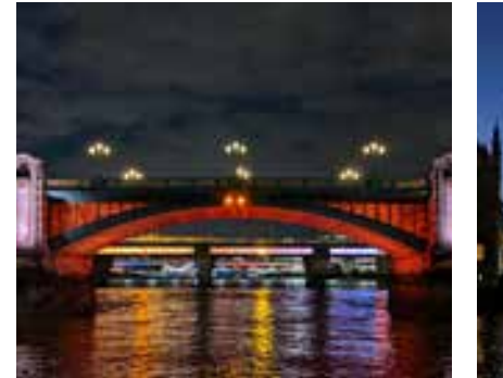
Image of Southwark Bridge
