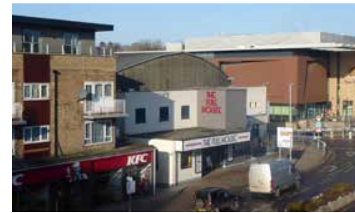
View of old cinema at the junction between Marlowes and Combe St
