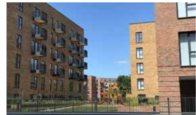
The Gade residential development located on the southern side of the Civic Zone site
