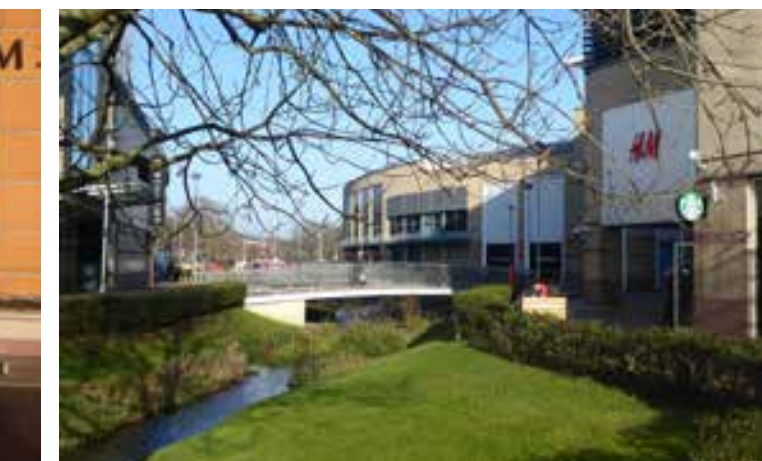
View of Riverside Shopping Centre from bus stop looking north
