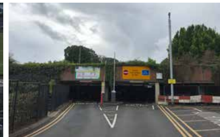
Entrance to the Water Garden Car Park North from Combe Street
