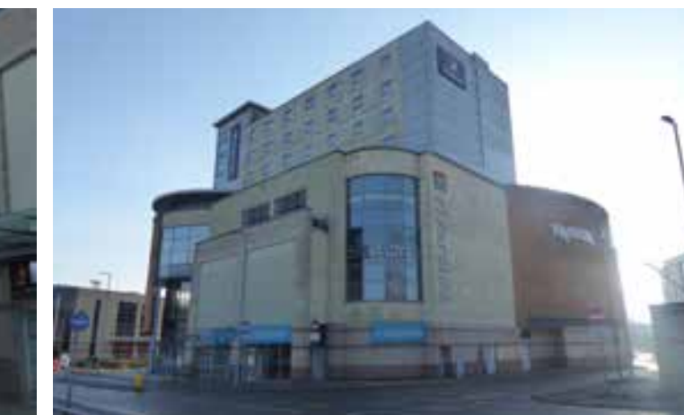
View of Riverside Shopping Centre from Moor End Road looking south
